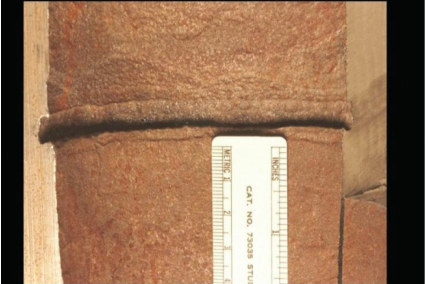
Figure 1.1. Preferential weld metal corrosion with some general attack on base metals
