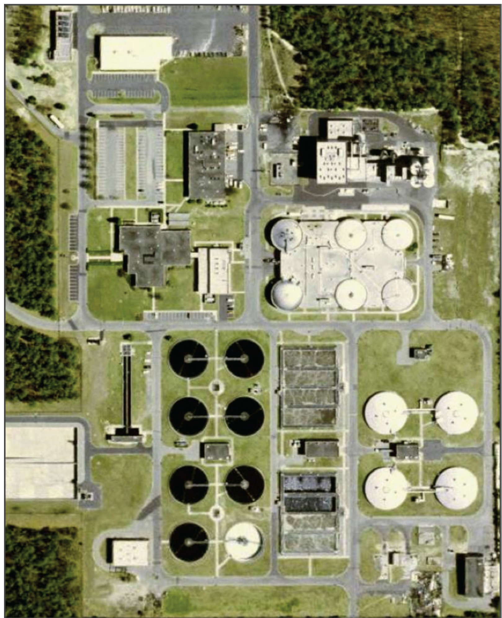
Figure 1. Aerial view of large wastewater treatment plant, showing circular clarifiers and digesters
